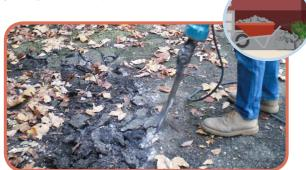
**De-Paving:** The removal of concrete, asphalt or other impervious surfaces can provide space for a lawn, rain garden, clean stone or other landscaping.
